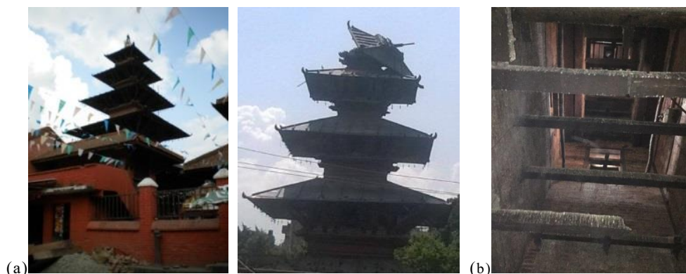
Figure 1 – Kumbeshwar temple in Patan, Nepal damaged/collapsed after the Gorkha earthquake: (a) Kumbeshwar temple.
